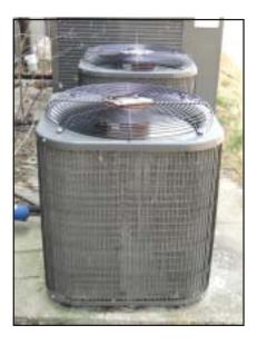
Standard 3½ ton condenser coil. Note debris in fins that can restrict air flow and add hundreds to power costs in a season.
