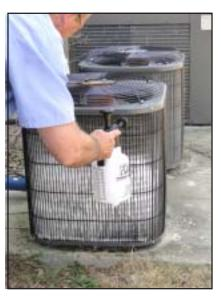
Con Coil applies in minutes. Foaming action removes corrosion and floats dirt and debris from the fins and coils.
